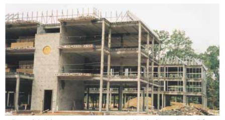
Hollowcore helped the Marriott meet restrictions on building height, providing a tall floor-to-ceiling room space on each level. Mechanical and electrical needs were run through the cores in the slabs to facilitate using the plank as a combined ceiling/floor.
